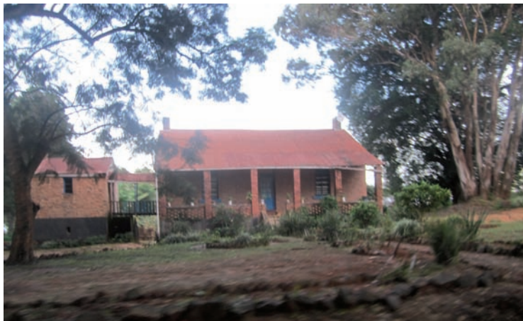
Mission houses. Typical design – made of brick and corrugated steel with outside veranda and kitchen attached through a covered walkway. This is the land of rain and damp enveloping cloud, and these are cold houses during winter-time.
