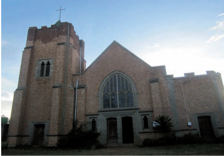
Christian Church. The church in all its glory as the original centre of Christianity in Northern Malawi and the catalyst for much of the social development that followed in the region during the ensuing 100 years.
