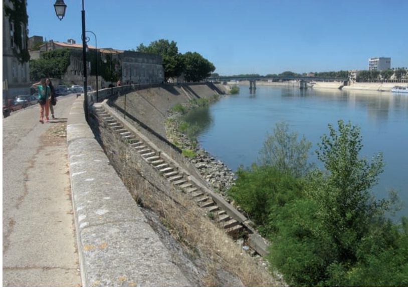
Rhone in Arles. Draining central France, but with low mid-summer flow the river is peaceful and unassuming. The retaining walls capture high flow in winter and spring. The main town is to the left and, across the steel bridge, the suburb of Trinquetaille – where the richer Romans once maintained second homes to escape the heat of the coast.
